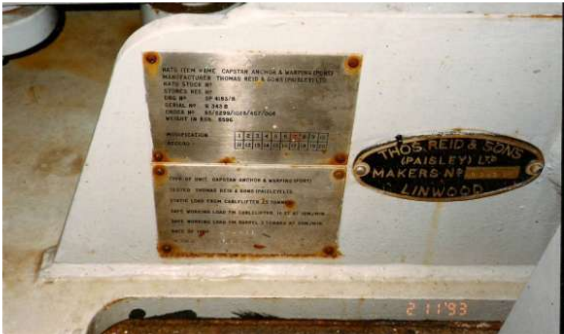
Figure 3.5 Manufacturers Nameplate with incorrect Fasteners
