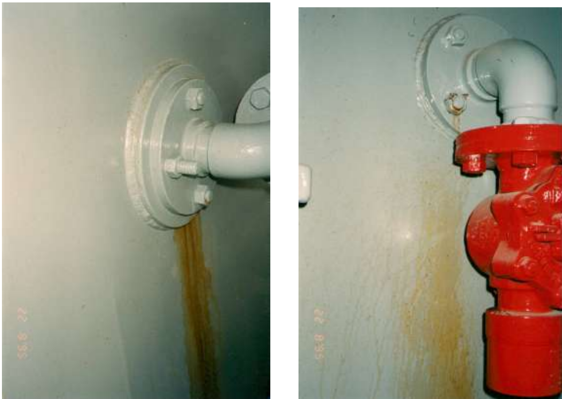
Figure 3.1 Rust Staining from Flange bolts
